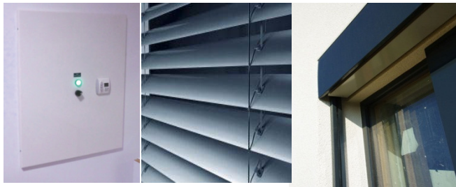
The last user switch off all the office area, before leaving by the end of the day, just by its single switch action.
